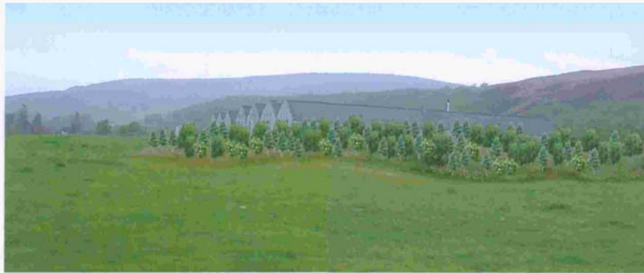
Eastern view of warehouses, with mounding and planting after approximately three years of growth.
