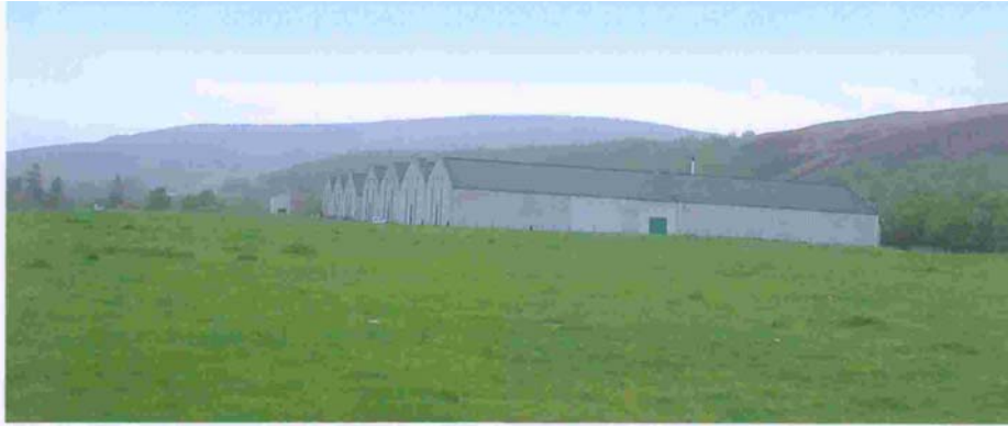
Eastern view of warehouses, with no mounding or planting.
